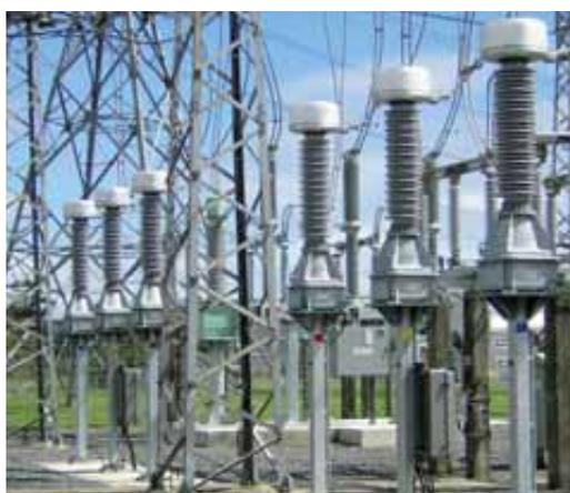
2. 123 kV Inductive voltage transformers. Transpower (New Zealand).
