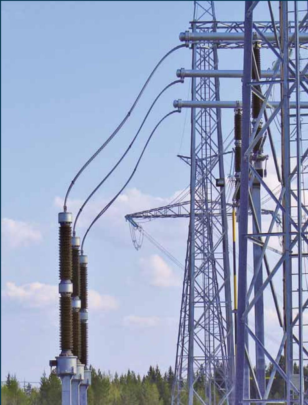
› 420 kV Capacitive voltage transformers. Fingrid, Visulahti (Finland).
