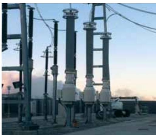
4. 420 kV Inductive voltage transformer. R.E.E. (Spain).
