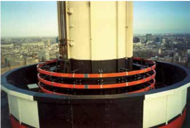
*Four closed curved tracks for feeding of a rotating elevator.*
